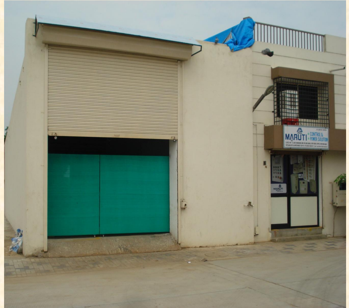
MANUFACTURING WITH FULLY TESTING FACILITY
